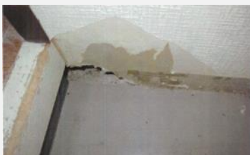
Wallpaper peeling off, floor damage
